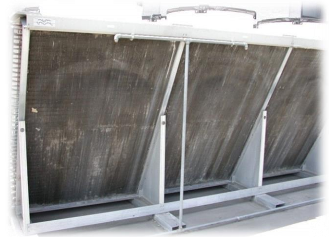
"V-shape" dry cooler after 1 year operation
